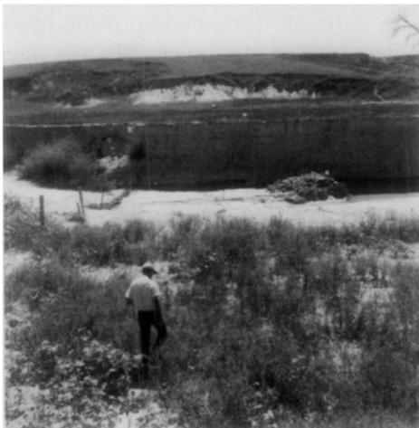
FIG. 7. Photographs of cross section 6 taken in 1957 (A) and 1967 (B). Over 2 m of sediment has filled in this cross section in the 14-yr interval between the 1957 and the 1971 surveys. Downstream is to the left in both photos.
